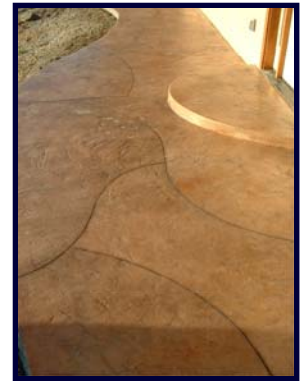
Stamped, stained concrete
